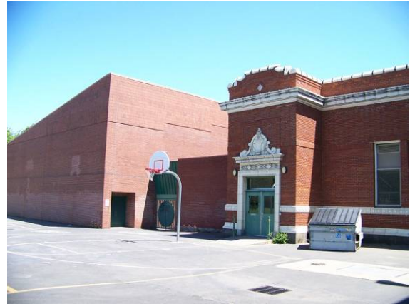
Main building (249A) and 1978 addition (249B), west (side) elevations, looking northeast.
