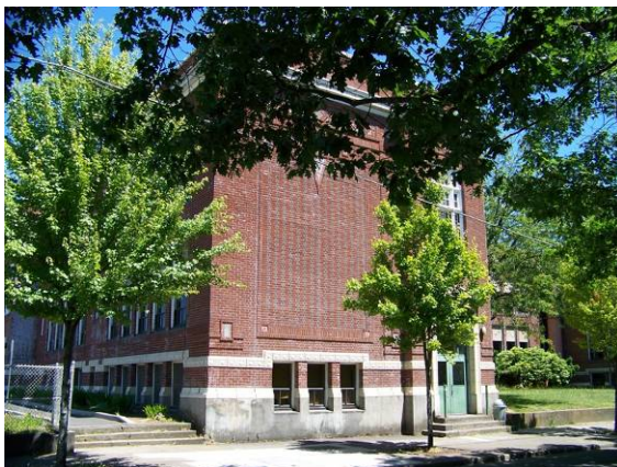
Main building (249A), south and west (side) elevations, looking northeast.
