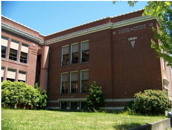
Main building (249A), south (original front) elevation, looking northeast.
