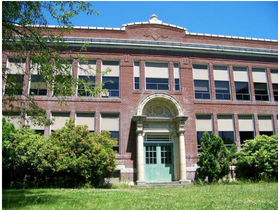
Main building (294A), south (original front) elevation, looking north.
