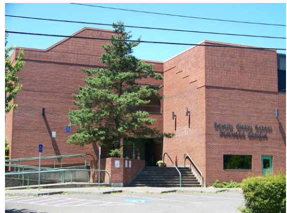
1978 addition (249B), east (front) elevation, looking northwest.
